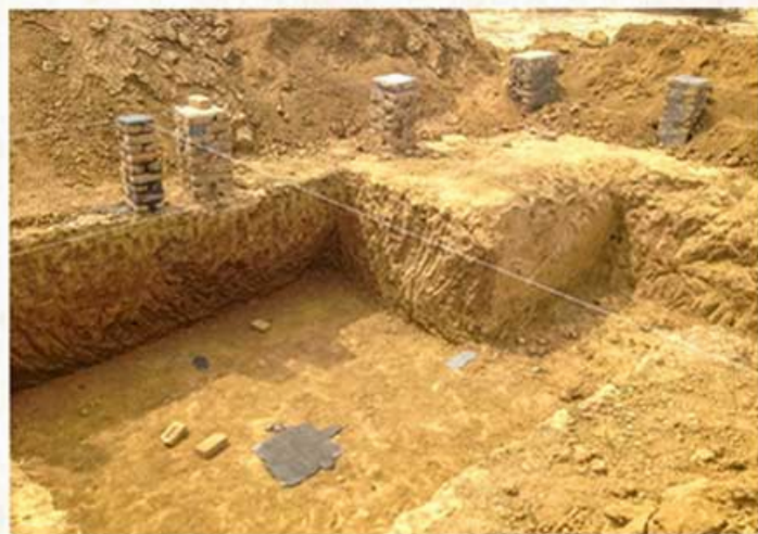
Construction started on 3 rd Feb, 2016
